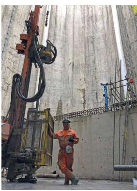
75m, then installed a 125mm wellscreen with filter pack. On completion of the well, a borehole pump was installed and a series of pump and recharge rate tests were undertaken as part of groundwater monitoring within the diaphragm walls of the shaft.
